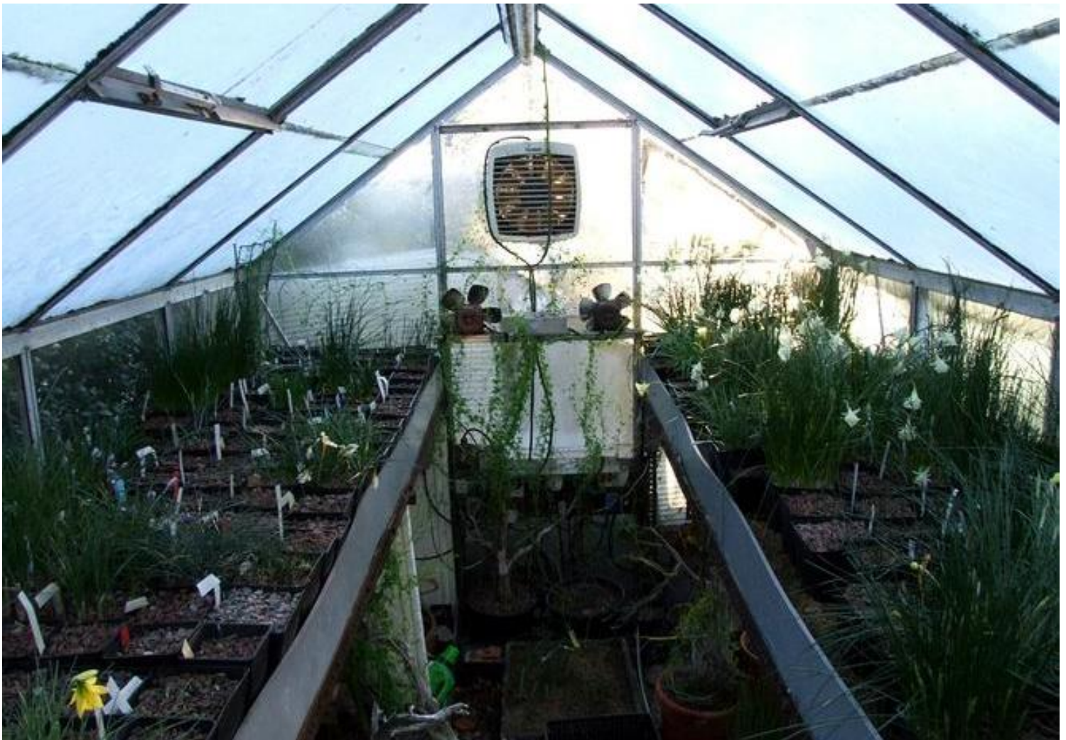
Frost inside bulb house
